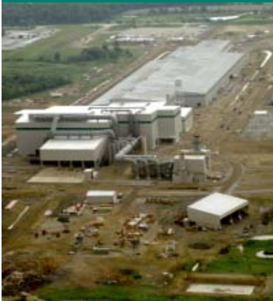
Aerial view of the SDI facility, looking west to east. The scrap-handling building and bag-house are in the foreground, with finishing facilities located in the background.
